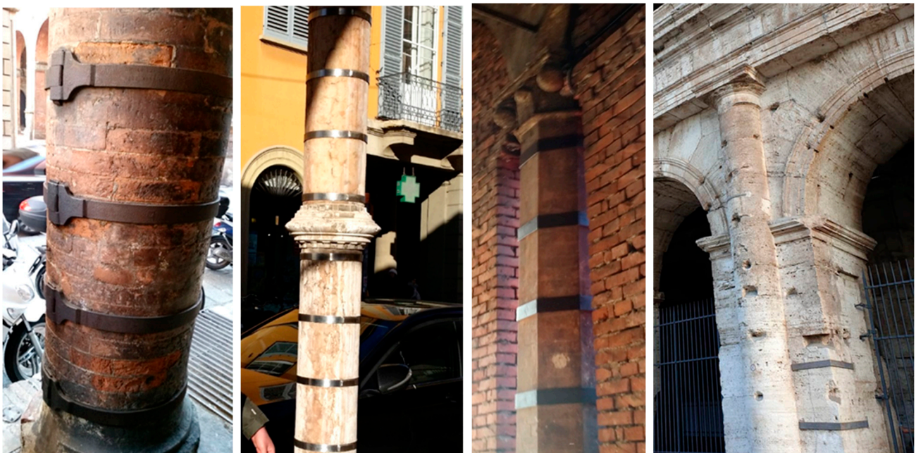
Figure 15. Brick and stone columns confined with discontinuous wrap configuration, Bologna, Italy.
