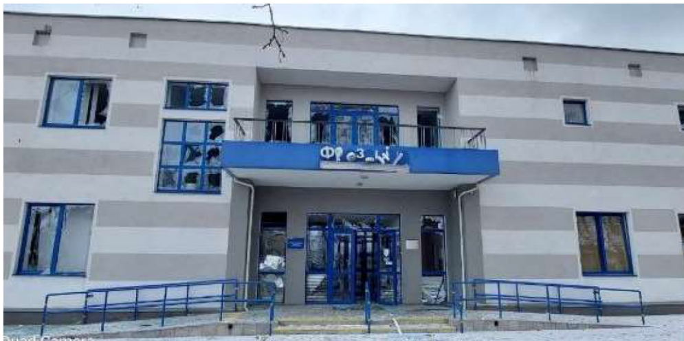
Figure 4: FME Chernihiv clinic damaged by a rocket attack.
