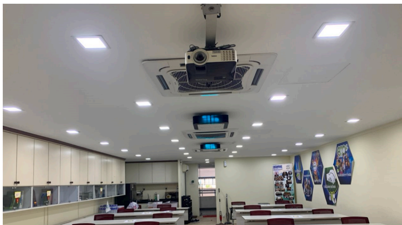
Fig. 5. Upper-room UVGI installed in an office in Malaysia.
