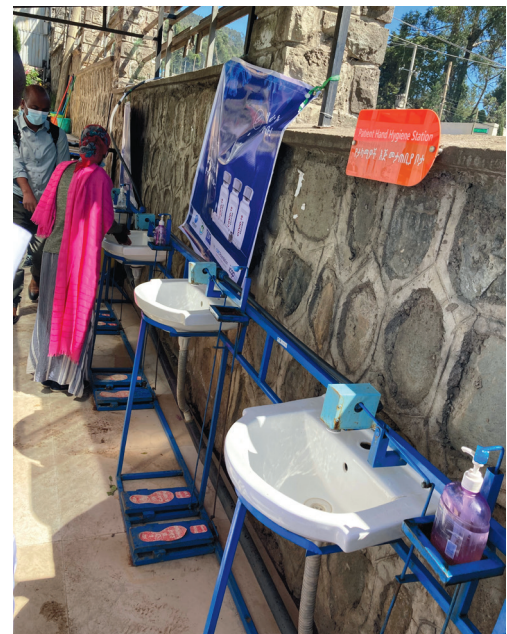
Photo: Patient handwashing stations installed at a healthcare facility in Addis, Ababa Ethiopia as part of the COSMIC project. Source: CDC Foundation, used with permission obtained from partners.
