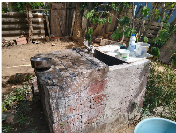
Fig. 3 A concrete ground tank for washing purpose
