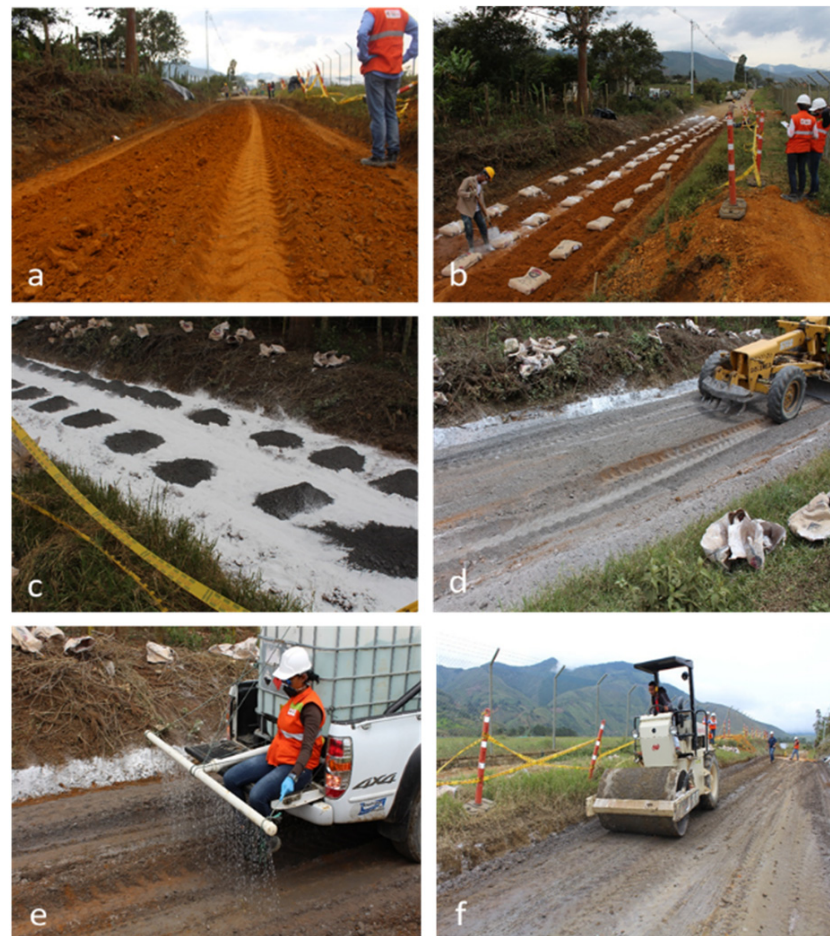
Figure 4. (a–f) Test track construction process.
