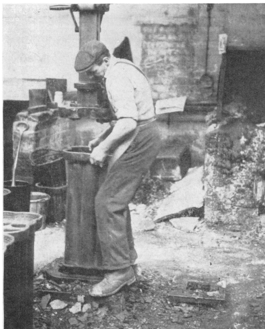
FIG. 3.—Handling the pipes on the lap.
