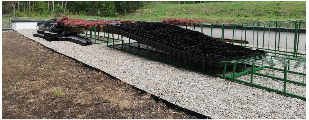
Figure 11. Welded mesh structures with differentiating heights.
