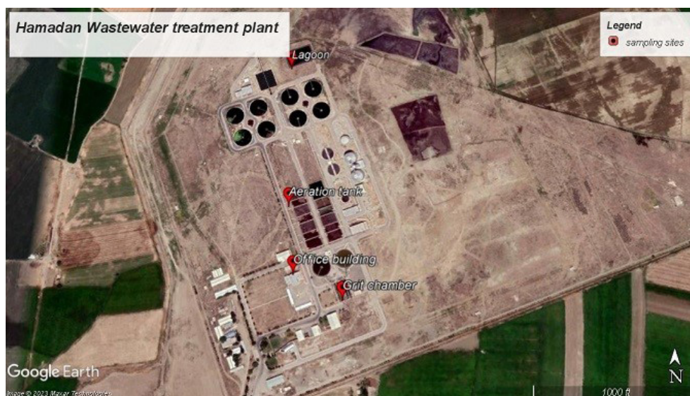
Figure 1. Sampling locations in Hamadan wastewater treatment plant
