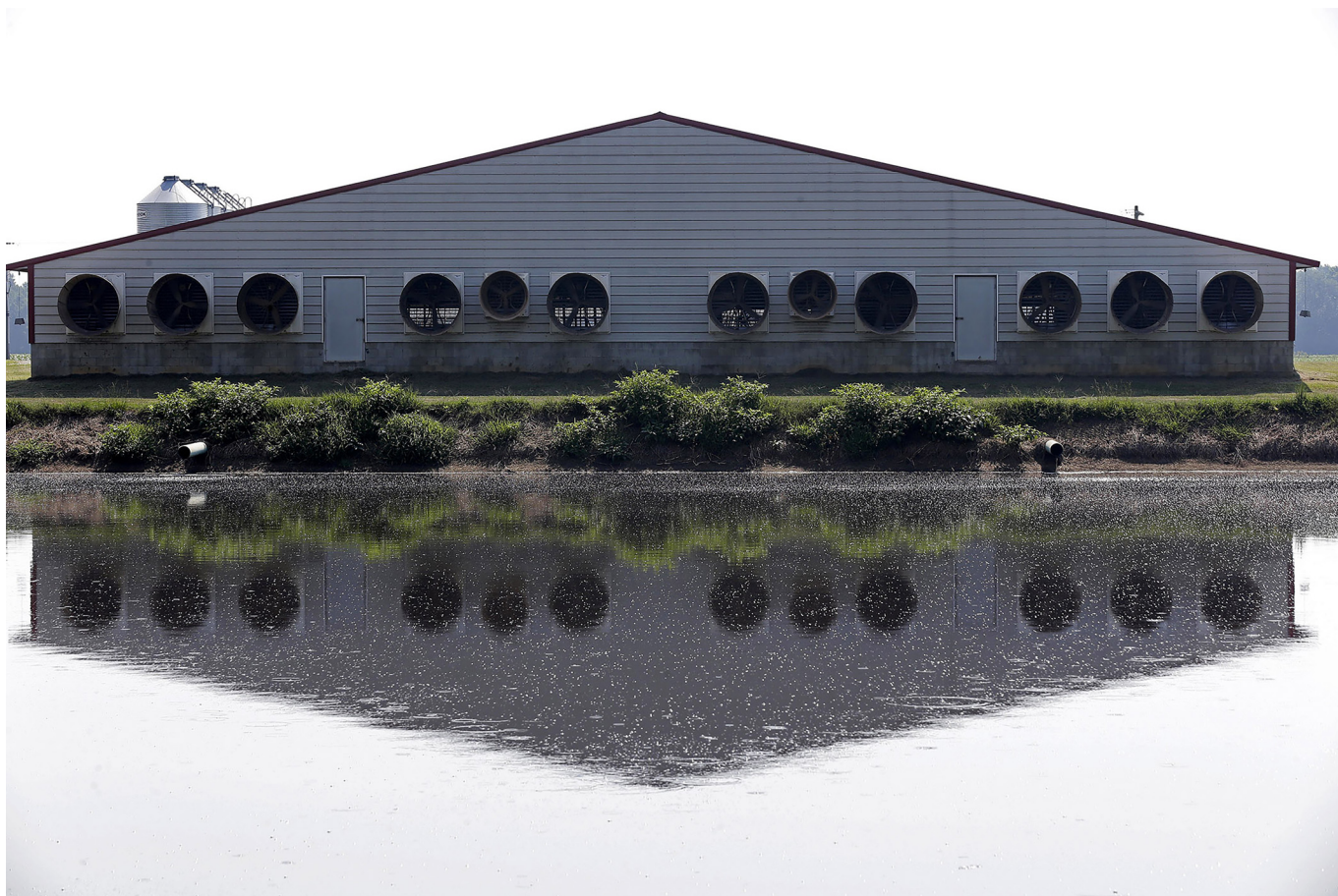
Hog CAFOs emit pollutants from waste lagoons, like this one next to a barn in Pitt County, North Carolina; in air exhausted from barns; and when wastewater is sprayed on fields. Image © Gerry Broome/AP Photo.
