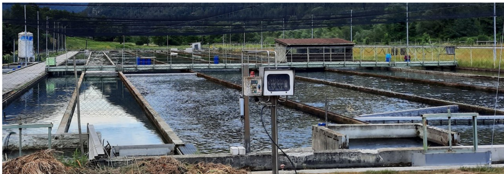
Figure 1. Raceway tanks, the liquid oxygen tank (white tank in the left) and the gantry (containing movable catwalk which crosses the raceways).
