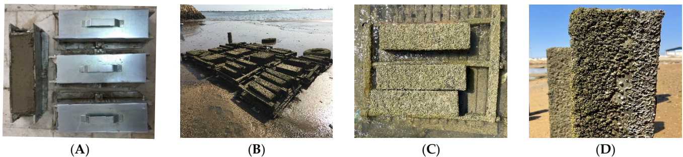
Figure 3. (A) Specimen molds, (B) Oman Sea tidal zone, (C) Tidal zone samples, (D) Specimens after leaving the tidal zone.
