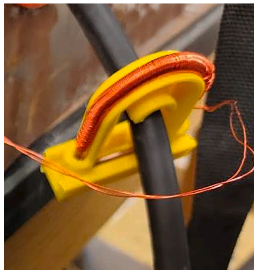
Fig. 44. A custom current transformer placed around the ground wire of the welder.
