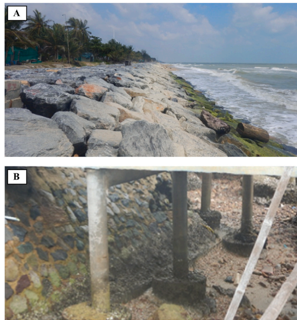
Fig. 5. A presence of benthic epifauna on revetment surface. (A) A rock revetment, and (B) a concrete revetment.
