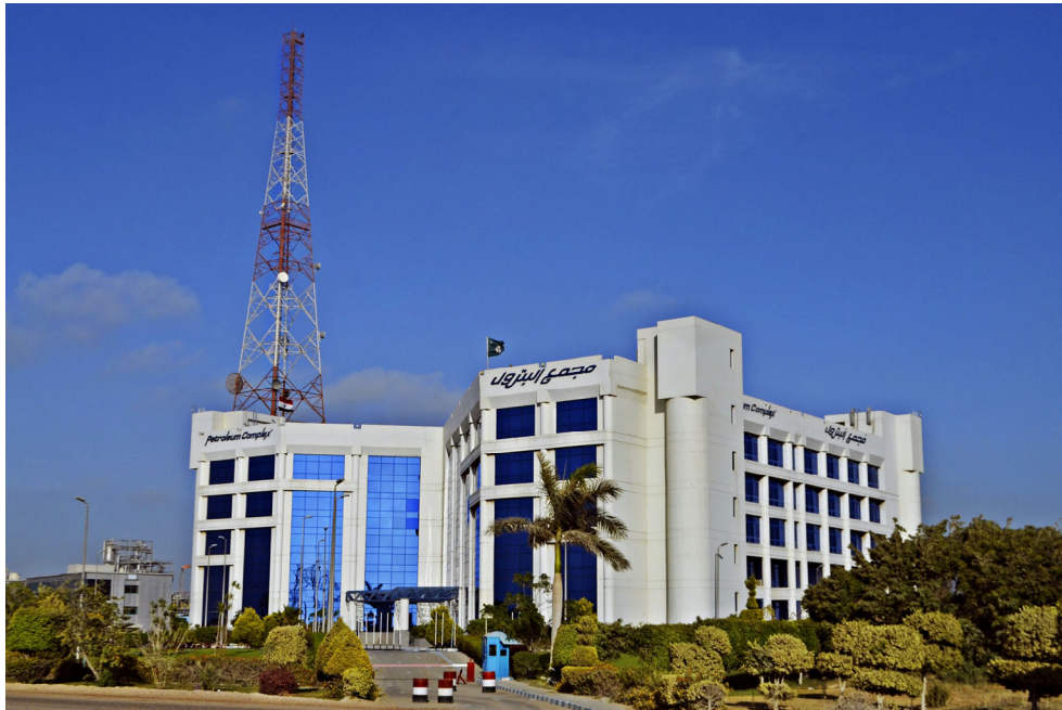
Figure 13. Cairo Petroleum Complex Building North-West main elevation showing the buildings Curtain wall façade: Wikipedia.
