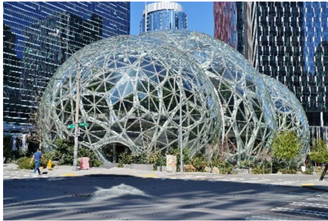
Figure 8. The Amazon Spheres three glass domes that are covered in pentagonal hexecontahedron panels: Wikipedia.
