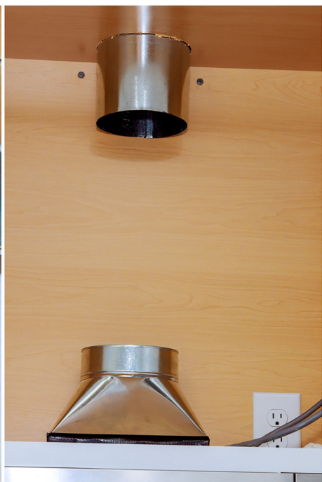
Using range hoods that exhaust to the outside, such as the one being installed above, and opening windows where feasible are ways to help reduce levels of harmful pollutants generated by even well-functioning gas stoves. Images: © Ungvar/Shutterstock.com.
