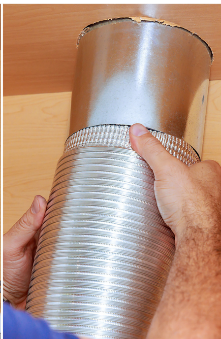
Using range hoods that exhaust to the outside, such as the one being installed above, and opening windows where feasible are ways to help reduce levels of harmful pollutants generated by even well-functioning gas stoves. Images: © Ungvar/Shutterstock.com.
