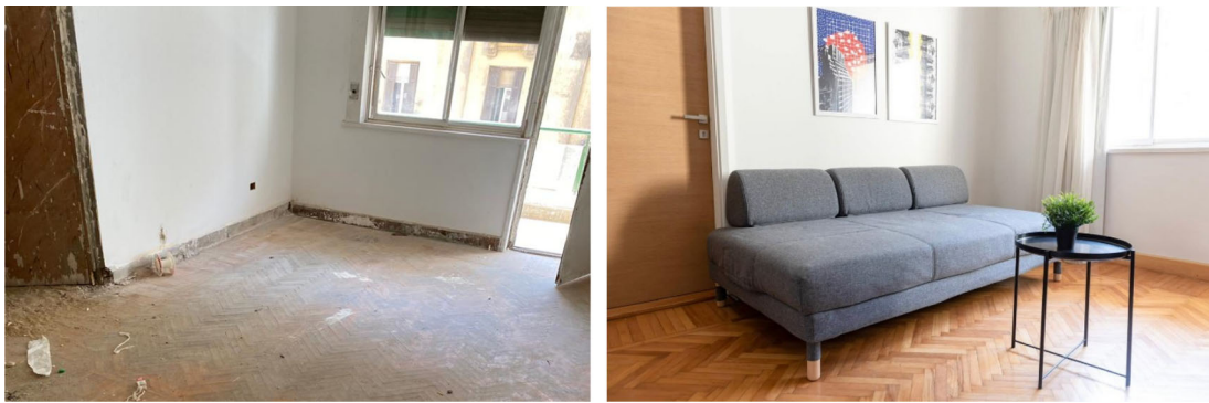
Figure 23. Before and after status of one of the units which had original parquet floors, those were restored and reutilized in the space, also another feature that was restored was the original windows and roller shutters. Source: This figure has been reproduced with permission from Sigma Properties, 2022.
