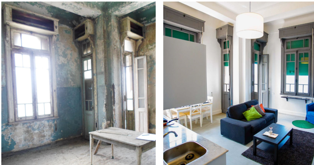
Figure 17. Before and after status shows how the existing elements were preserved such as the wooden doors and windows, and the original roller shutters in order to preserve the building's identity and unique heritage significance. Source: This figure has been reproduced with permission from Sigma Properties, 2022.
