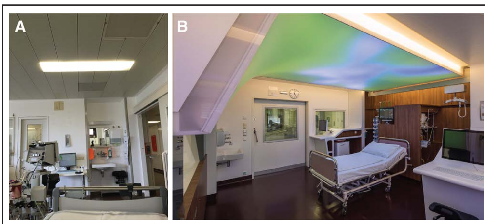
Figure 1. Pictures from one of the two-bed-rooms on ICU-8i at Charité Campus Virchow-Klinikum before (A) and after (B) the architectural and design modifications. The light-emitting area of each dynamic lighting system covers a surface of up to 6.1 \text{ m} \times 2.4 \text{ m} for one ICU bed.
