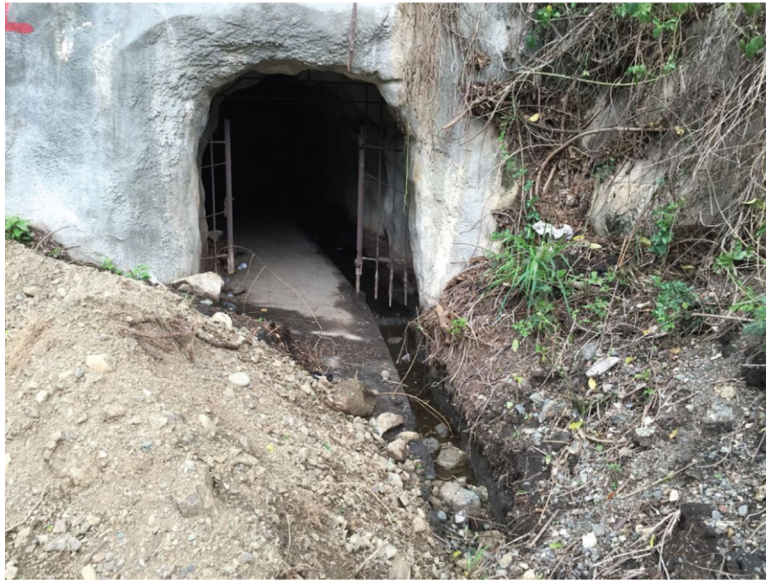
Figure 1. Entrance to a tunnel associated with severe histoplasmosis outbreak, Dominican Republic.
