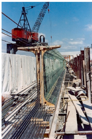
Fig. 1. Pre-tensioned bridge girder in casting bed, with single-strand tendons placed in the formwork [67].
