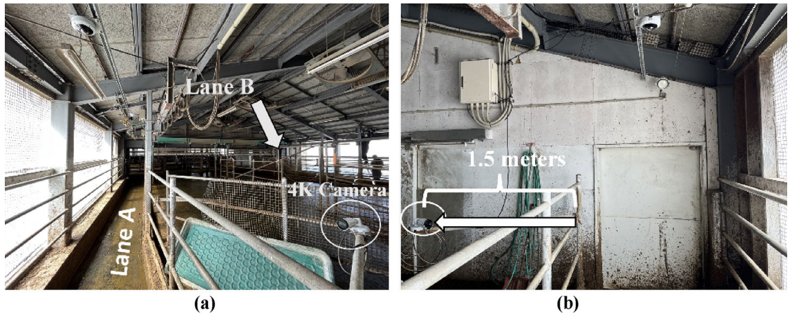
Figure 5. Camera installation (a) 4K camera on lane A (b) front-view from 4K camera installed.
