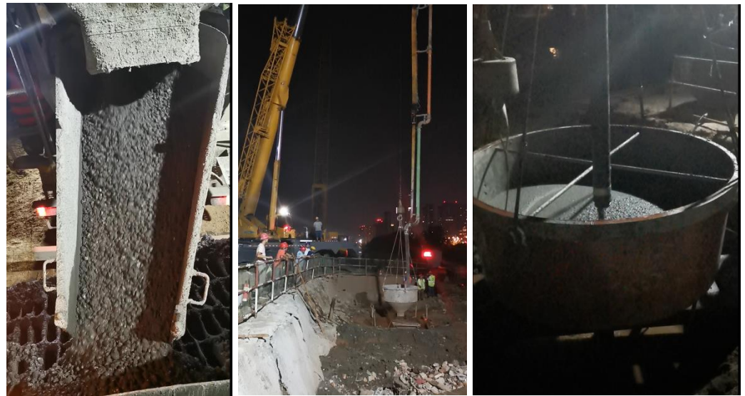
Figure 9. Onsite pumping and placement of concrete.
