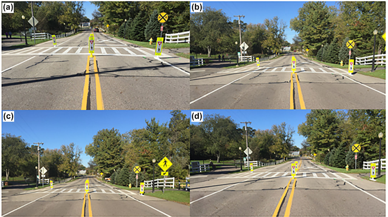
Figure 3. Gateway widths of (a) 12 ft, (b) 14 ft, (c) 16 ft, and (d) 18 ft.
