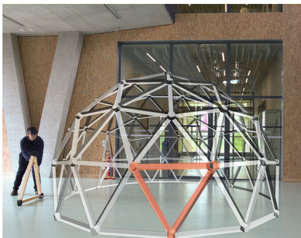
Fig. 10 | Using XR for the structural assembly of a dome with reclaimed elements.
