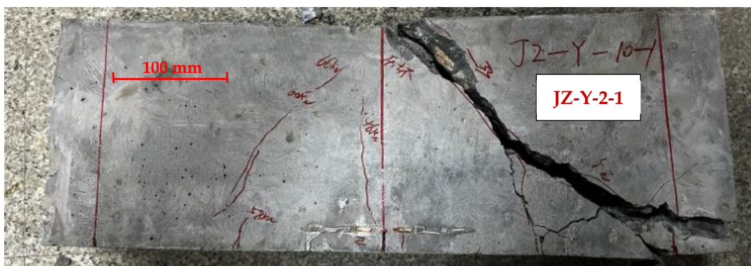
Figure 11. Side view of a typical fractured reinforced concrete specimen. Besides cracks initiated from the prefabricated notch, oblique cracks were also developed, eventually leading to anchoring failure. Please note that a label was added to the picture because the specimen was initially named after the notch-to-height ratio of 0.1.
