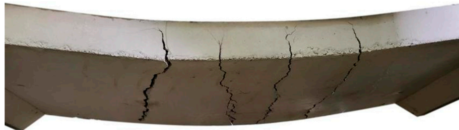
Figure 12. Cracks and the failure mode of the control slab.
