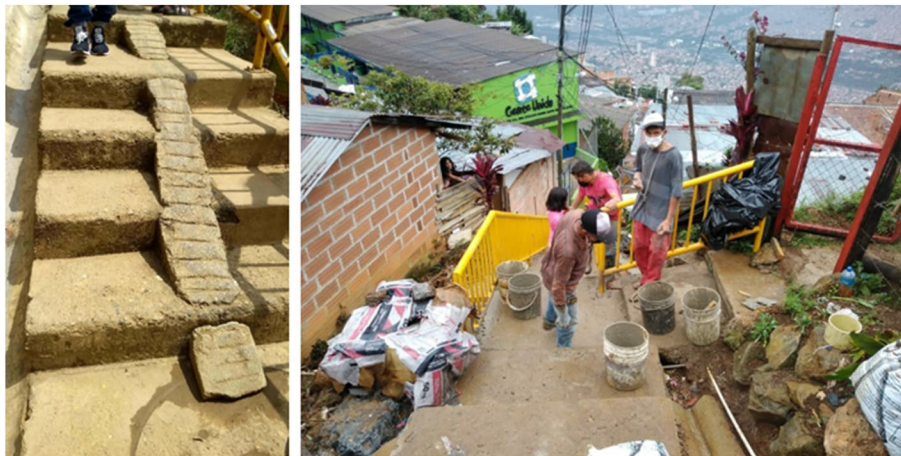
Fig. 4 Communally built steps with ramps for motorbike access in IDP settlements. Source: Photo taken by one of the authors
