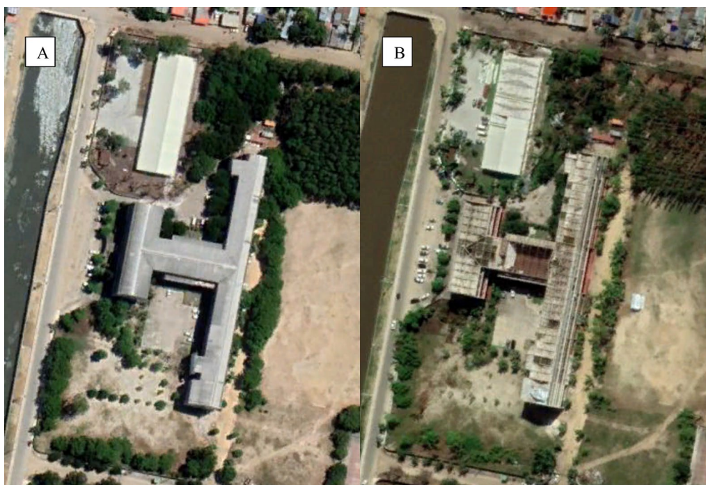
Fig. 2 Pre and Post Cyclone Imagery of University in Beira, Mozambique. Image A is taken from satellite imagery in March 2019 prior to Cyclone Idai. Image B was taken in April 2019 immediately following the cyclone. Here there is clear evidence of complete damage to this facility following the storm
