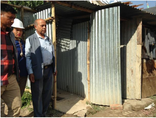
Photo 4. A toilet was built in a small construction site responding to the proposal of women construction workers.
