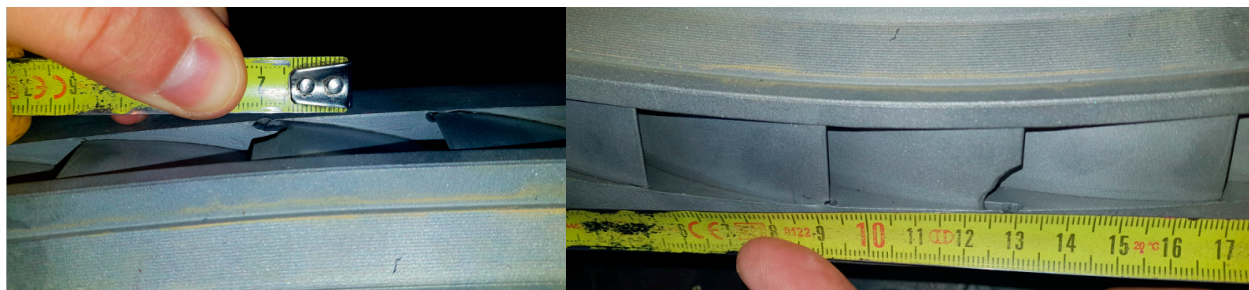
Figure 3. View of the new segment's nozzle with a close-up of the exhaust side after 22 h of operation. Nozzle boxes removed from the turbine.
