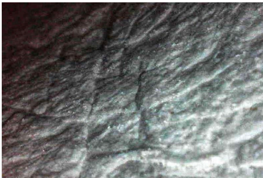
Figure 20. Cracks formed at the impact of hole 2.
