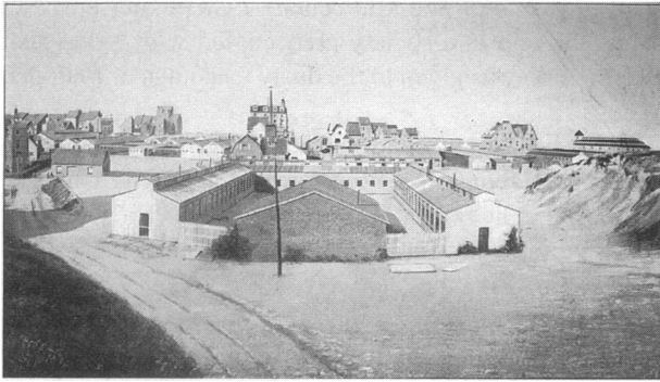
Figure 2. Depage's Ambulance de l'Océan, or military hospital, at La Panne on the North Sea, 10 km southeast of Nieupoort and 12 km behind the trenches. The view is looking out to sea. In the foreground, the quadrangular buildings are the research facilities, renamed the Institut Marie Depage after his wife's death aboard the Lusitania . (Depage, A Ambulance de l'Océan a La Panne ).
