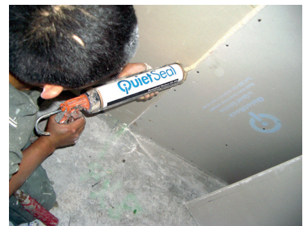
Caulk for quieter walls. New drywall and caulk are engineered to muffle building noise.
