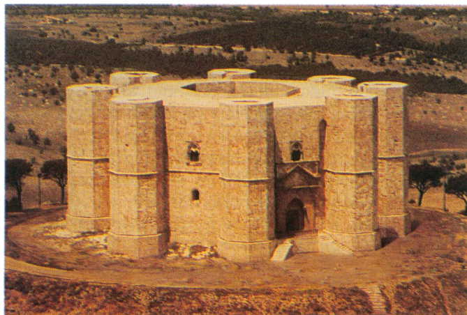
PLATE 10 Castel del Monte (Apulia, Italy), which has an eight-fold structure around a central opening and eight outer towers, each containing a right-handed spiral stair. Photo courtesy of Kasper Kirschner.
