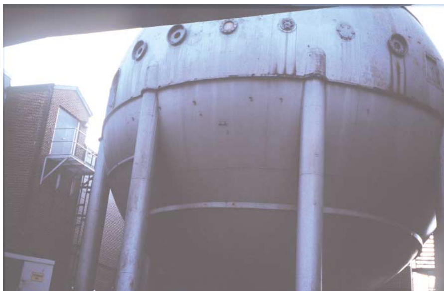
Fig. 2 | The so-called '8-ball', a 1 million litre steel ball built in 1949 in which the US Army tested the effectiveness of biological weapons. The ball is in Fort Detrick, Maryland, and is a 'historical monument' today. (© (2001) Jan van Aken/Sunshine Project.)
