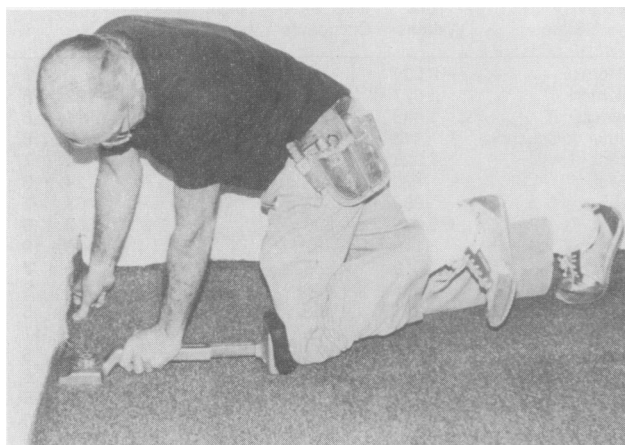
FIGURE 1—A Carpetlayer Using a Knee Kicker
