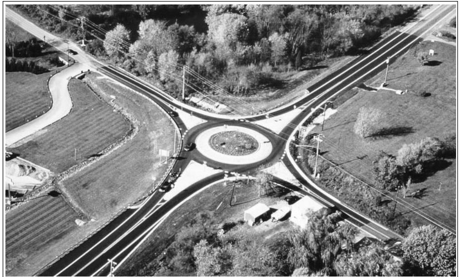
FIGURE 1—View of a roundabout in Cecil County, Md.
