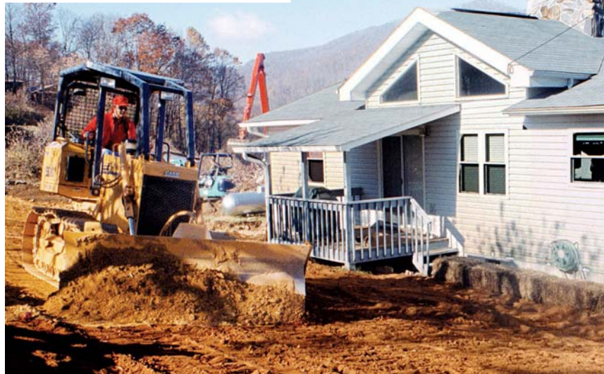
Landscaping. A bulldozer scrapes a layer of contaminated soil from a yard in the Barber Orchard subdivision in North Carolina, once the site of a large apple orchard. Due to contamination with former agricultural chemicals, the subdivision was designated a Superfund site in 2001. EPA-supervised cleanup, mainly by removing soil, is on hold pending further funding.
