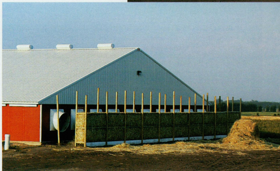
Just between phew and me. Exhaust air from hog barns is forced through barley straw biofilters that absorb both odors and dust.
