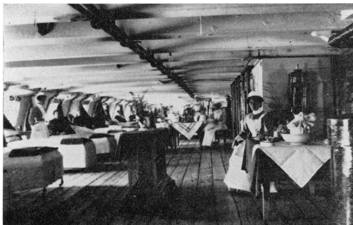
Fig 4 Ward deck on the Atlas. The rings for the gun chains can be seen above the beds. Headroom is 7 ft (2.13 m)
