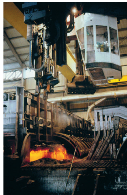
Figure 4 Overhead crane in pre-bake potroom.
