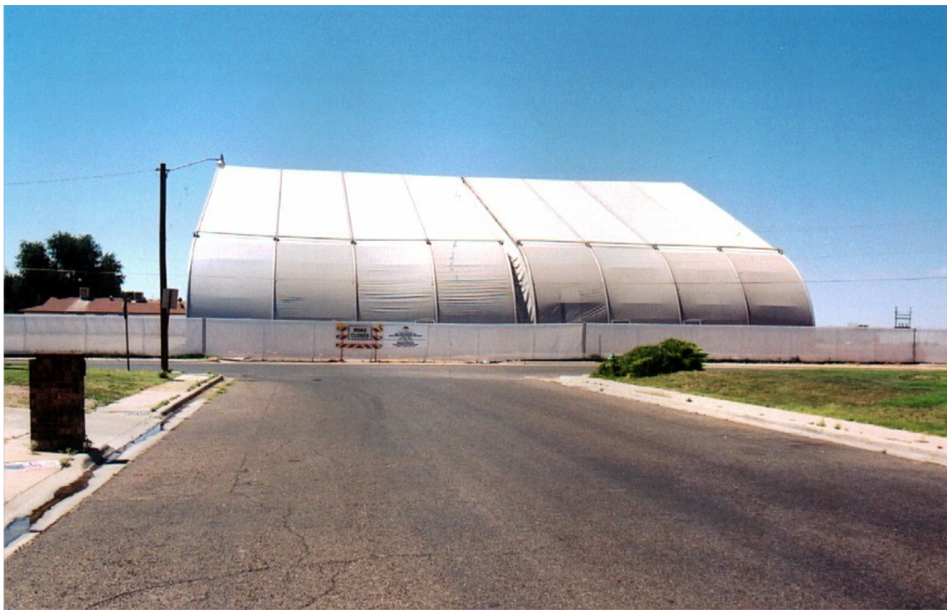
Figure 3 Close up Photograph of Tank Battery in Relation to one of the two exposed Streets.
