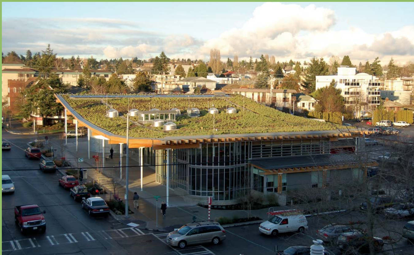
The Ballard Library in Seattle incorporates solar panels into its green roof design. Energy generated from these panels is fed back in to the city's power grid. The curved roof create six microclimate conditions, each a separate exposure with differing water retention properties, based on slope and orientation.
