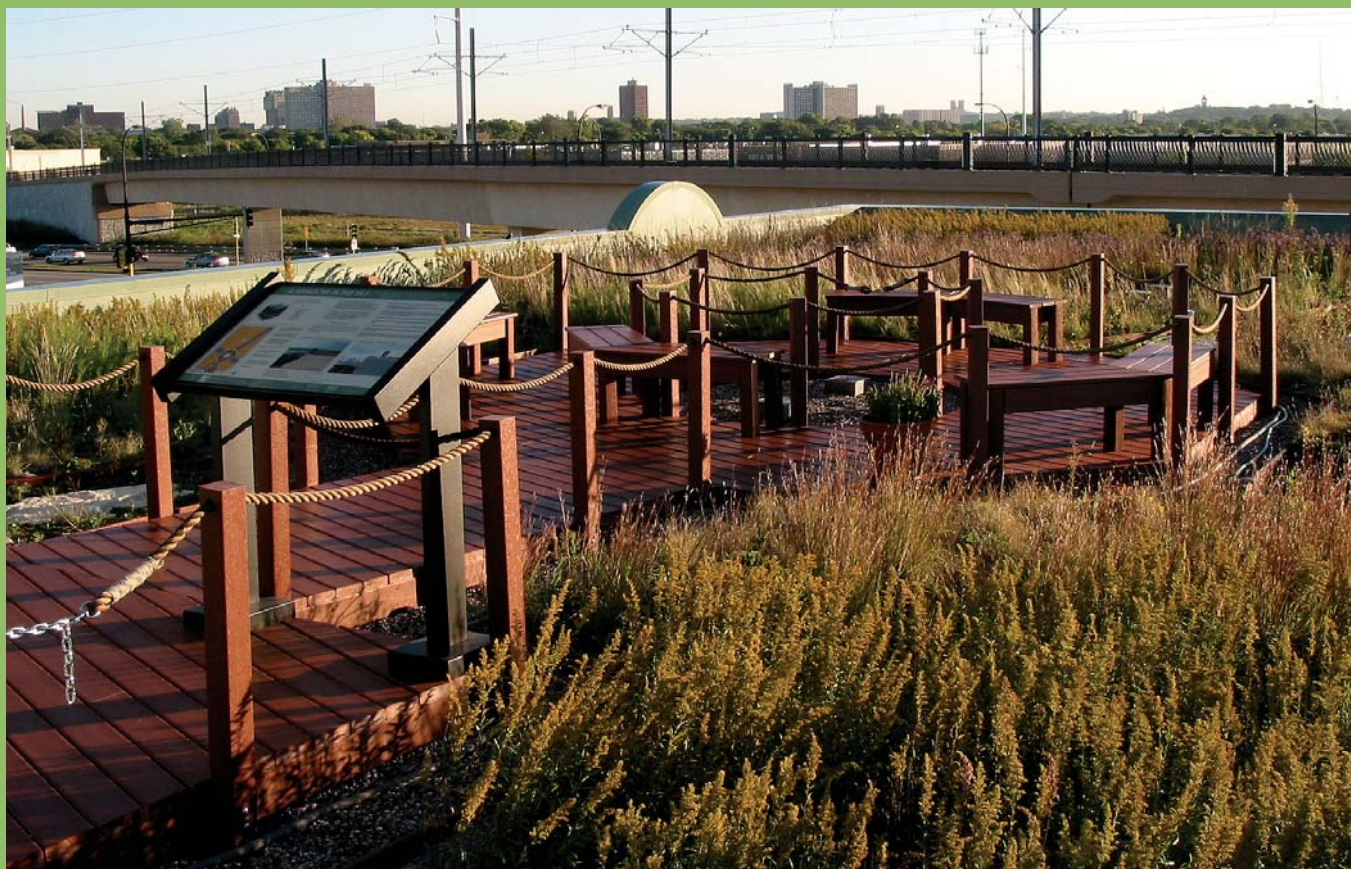
The green roof on the Phillips Eco-Enterprise Center in Minneapolis, stocked with native plants, educates visitors about the diminishing local bedrock bluff prairie ecosystem. The roof also offers a pleasing view to passengers on the nearby elevated train.
