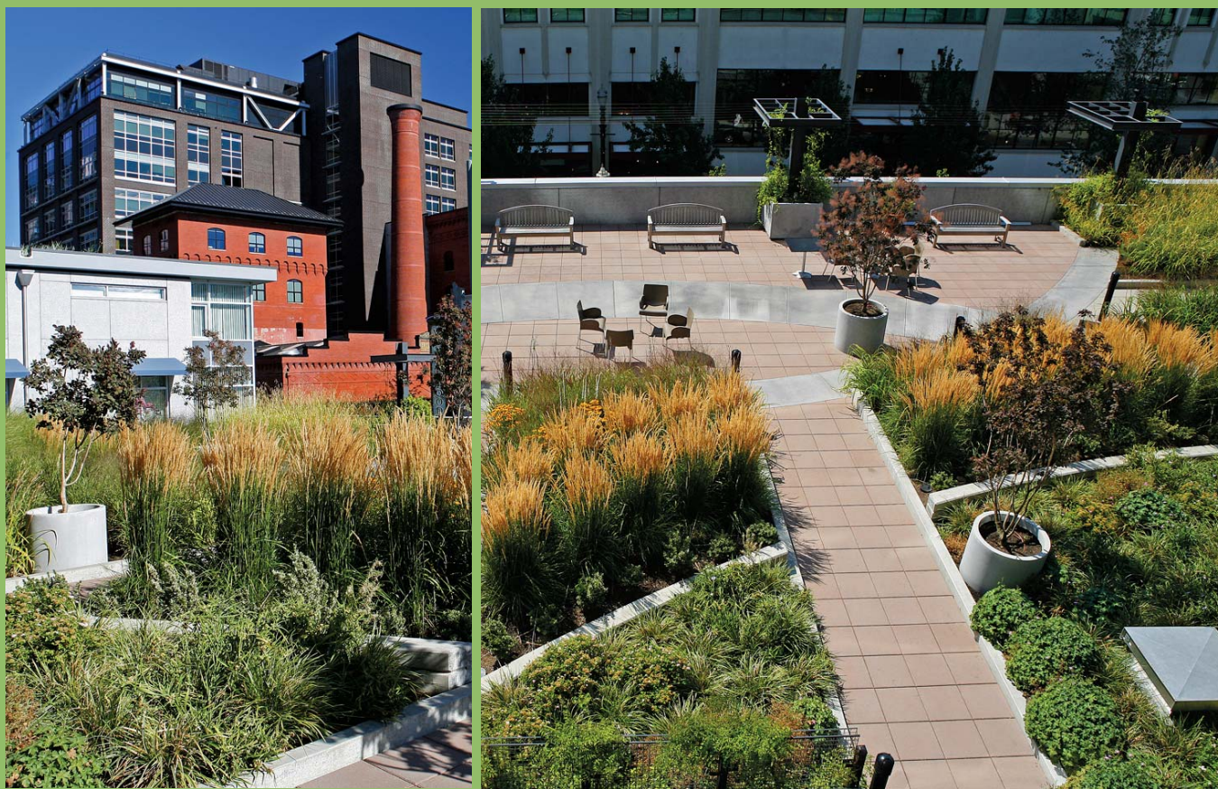
Two views of the Louisa, a Portland, Oregon, residential high-rise with 242 apartments and ground-floor retail. Other green features of the building include high-efficiency glazing, low-toxicity building materials and finishes, and locally sourced construction materials.
