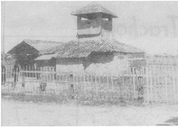
Blockhouses built of adobe bricks, such as the one shown here, or of thatching are located throughout the delta. The villagers in the surrounding area gather in these houses for the night.
