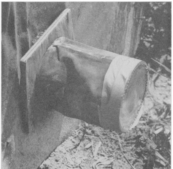
Closeup of fly trap on exterior of privy.
