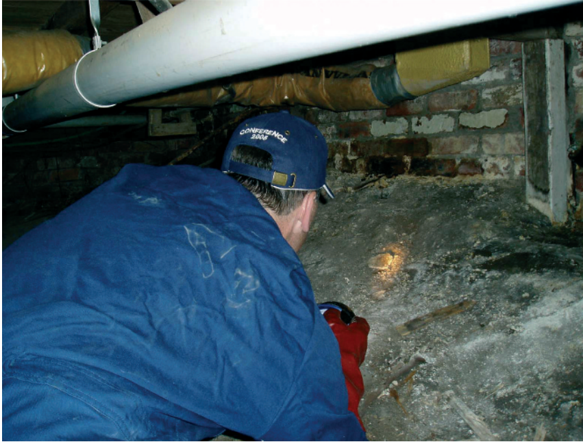
Figure 3 Accessing under-floor space.
