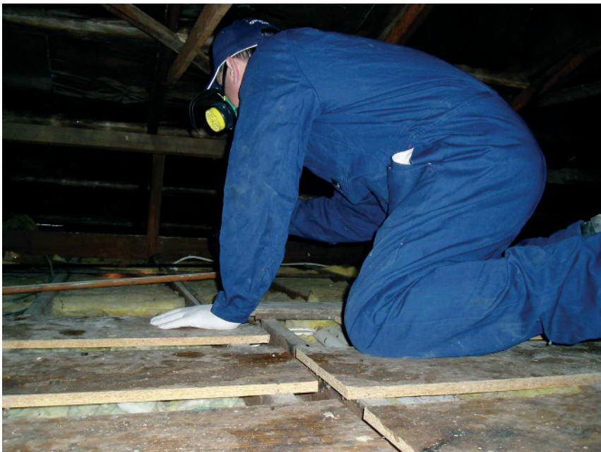
Figure 4 Accessing roof space.
