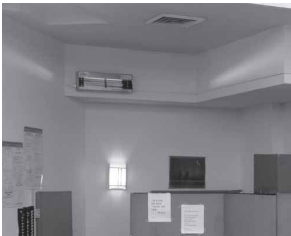
Louvered upper-air ultraviolet germicidal irradiation in Tuberculosis Ultraviolet Shelter Study New York City shelter. Photo: ©Randall Perry Photography.
