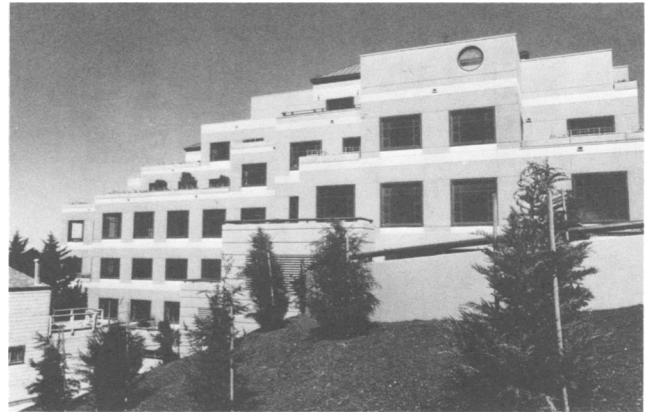
Figure 1 West facade, UCSF library (photograph by Deborah Stinski)
