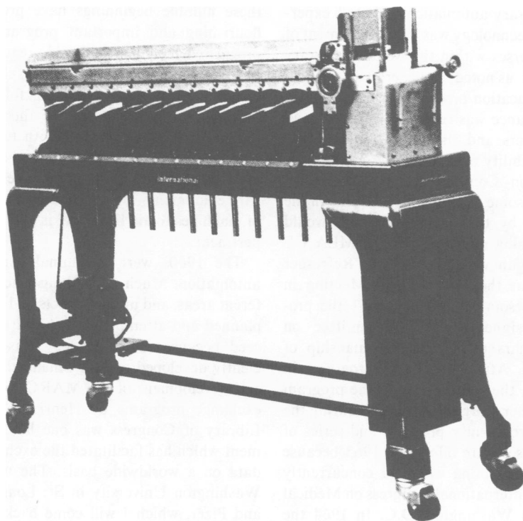
FIG. 4.—IBM card sorter, 1925.
